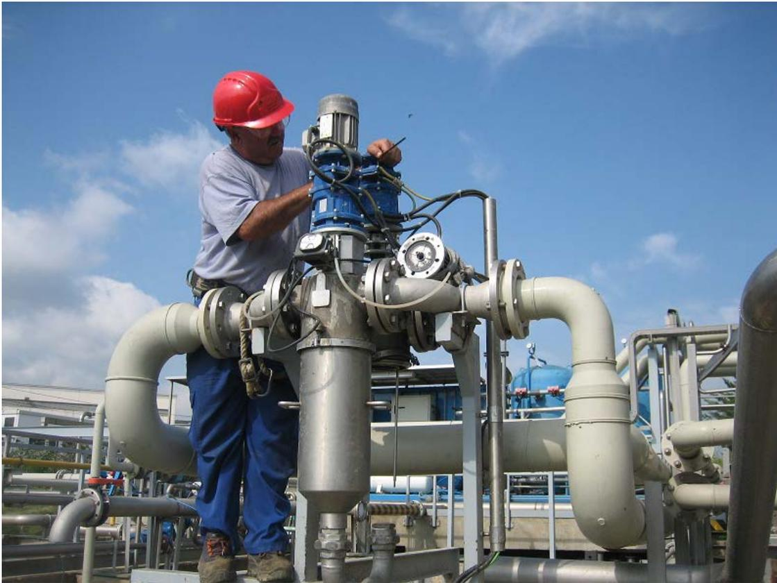
Self cleaning filters are easy to place and install. They can be placed in any section of horizontal pipe with liquid impulsion.
